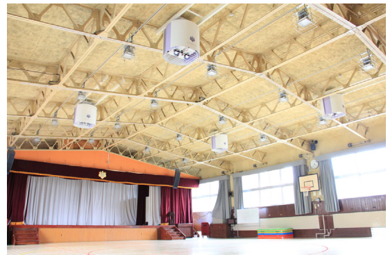
Fig. 3. Digital light processing (DLP) projectors and cameras on the ceiling of the gymnasium.
